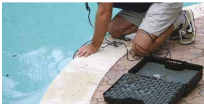
Leak detection, and Rectification
