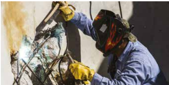
Structural Crack Pool Repair Service
