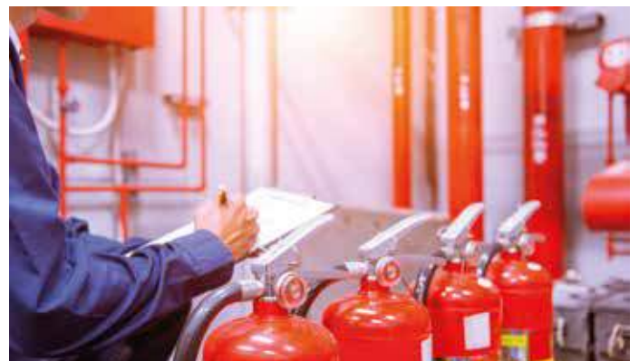
Fire Fighting – Installation and Maintenance
